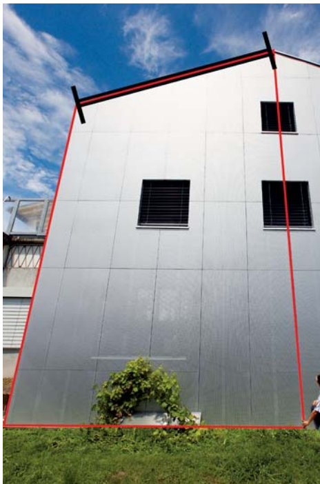
The trapezium function provides you with a simple way of measuring roof slopes.
